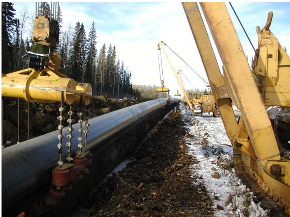
**Figure 4** Lowering in of pipeline.
