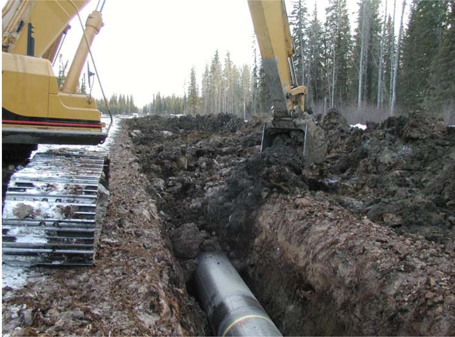
**Figure 5**      **Backfilling of pipeline.**
