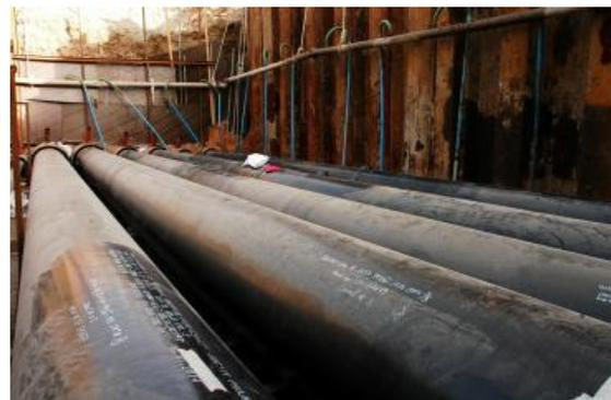
Figure 12 No damage of the new coating system was observed during field stencilling
