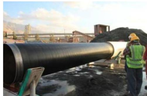
Figure 8 No holiday damage was detected at 20 Kv on the new coating system after concrete impingement
