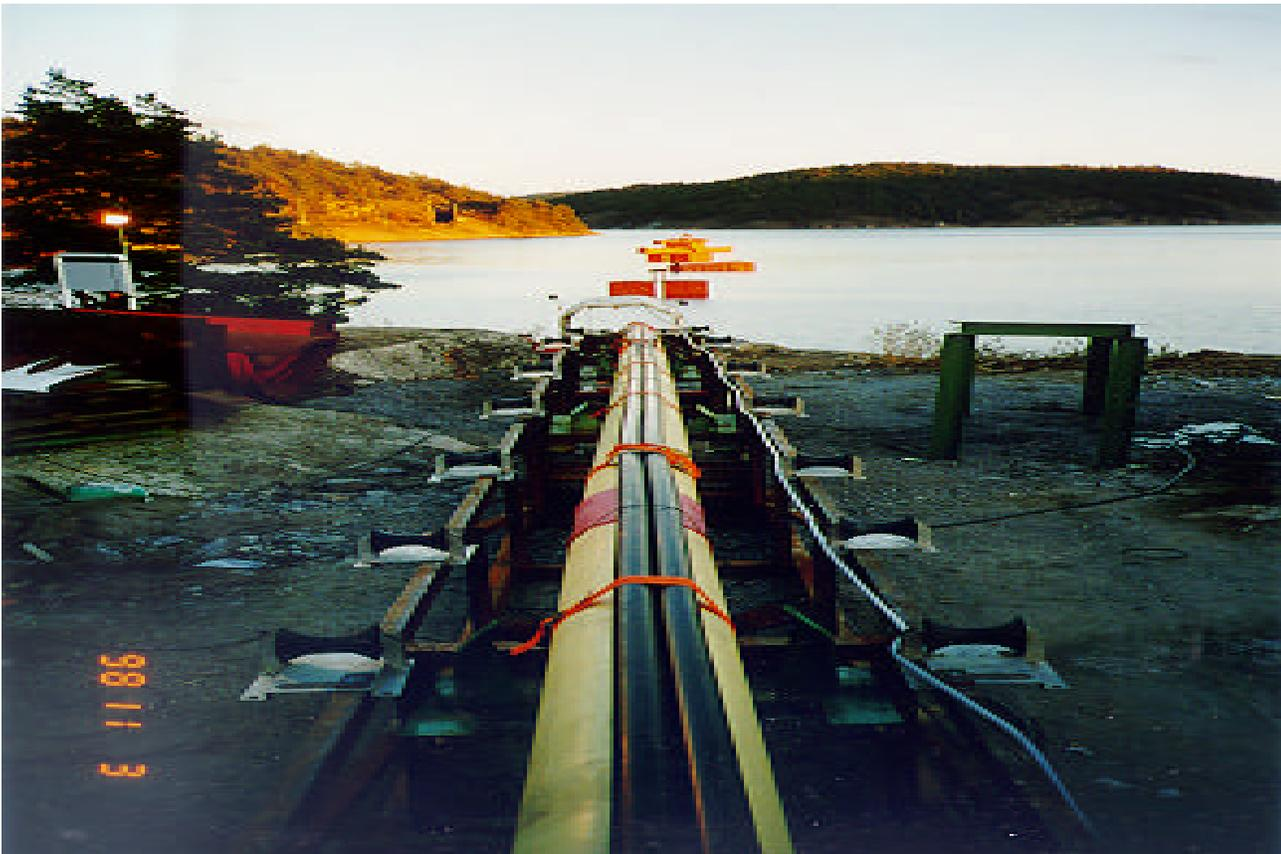
Figure11-Installation of field test flowline section (380m long)
